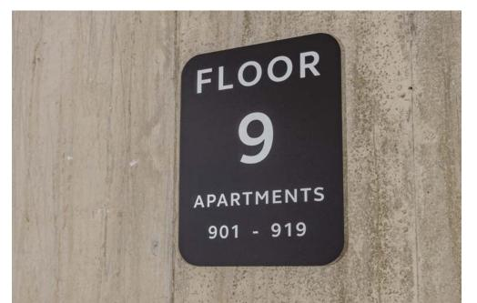
We have manufactured 3mm frosted slate grey Perspex signage through the stairwells to provide wayfinding. The directional signage is fitted to the substrate on spacers and secured with strong tape.
