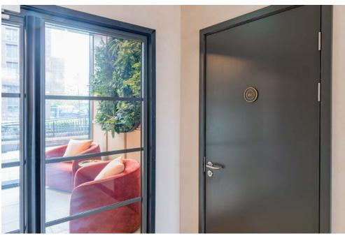
WC Toilet signs have been supplied using frosted grey panels with 10mm thick aluminium milled frames and painted Verometal detail.
