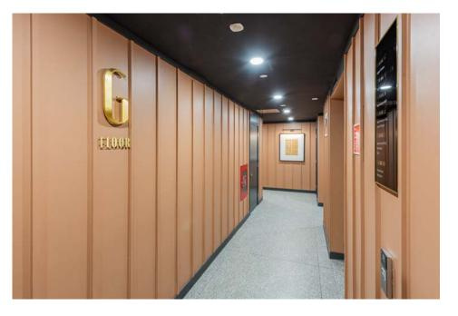
Floor level indicators are featured throughout the building. Gold leaf has been hand applied to mounted prismatic carved letters, spaced 10mm from the wall using brass tubes and spacers.
