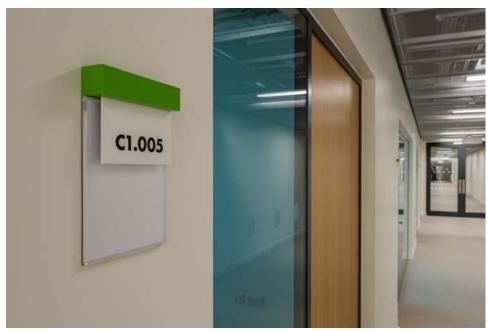
We have provided a bespoke modular signage system using a fabricated support bar to hold a suspended aluminium panel. A wall mounted Folio panel sits agaist the wall, with hidden mechanical fixings to ensure a secure connection.
