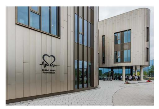
The external signage features 3mm thick aluminium, coated and applied with high grade paint and protective lacquer to preserve the finish.
