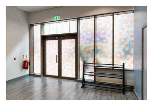
Digitally printed, profile cut dusted manifestations provide privacy. The client specified use of the Einstein shape as part of the design, to create a unique, non-repeating pattern - another reference to the purpose of the school.
