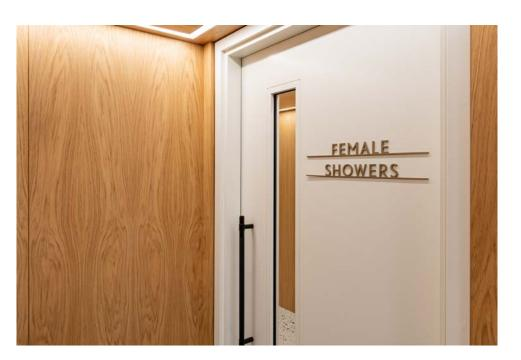
Cut letters are fixed above 3mm thick aluminium bezels to provide the appearance that the signage is sitting on a rail.
