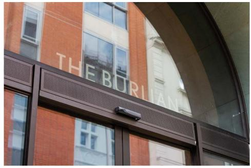
On entrance to the building we have provided 4mm thick aluminium letters with a ground and smoothed finish. The letters feature a folded base to allow for screw fixings to the canopy.
