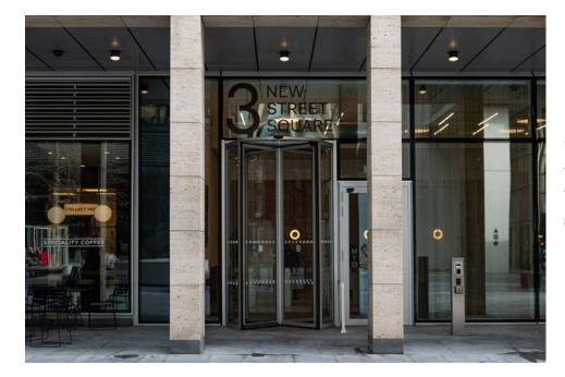
The external aluminium lettering features a ground and smoothed edge finish with face coating and a high grade painted finish.
