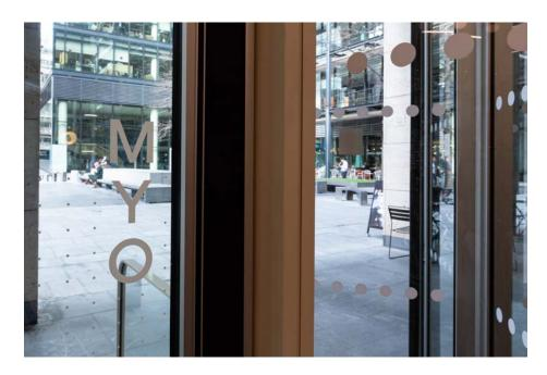
We've provided white UV printed optically clear manifestations as per the clients branding requirement. Additionally, dusted dots provide a key safety element required for glass doors and walls.
