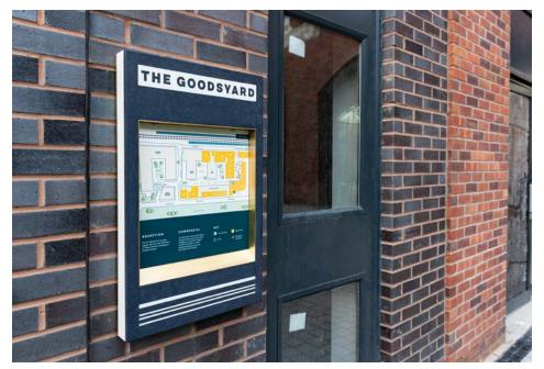
The wall-mounted map directories are made from an aluminium framework, custom painted aluminium faces, Corian Cameo White returns and satin brass return trims. The face of the sign has a Corian header, with custom painted blue lettering.
