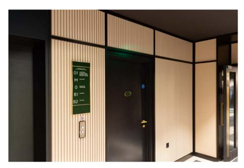
Aluminium base panels with brass frames feature throughout the living spaces to complement a high end finish.
