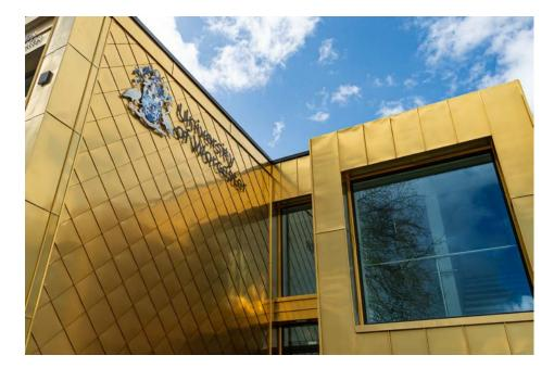
The external logo signs use intricately cut 4mm aluminium sheet metal with vinyl in-fill and lacquered weather protection. The aluminium cut letters are fixed with 25mm spacers to provide a 3D effect.
