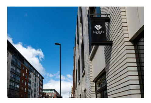
Double-sided illuminated LED projecting sign with brass detail and cut vinyl graphics. Clad with aluminium panels and top/bottom access caps for cabling.
