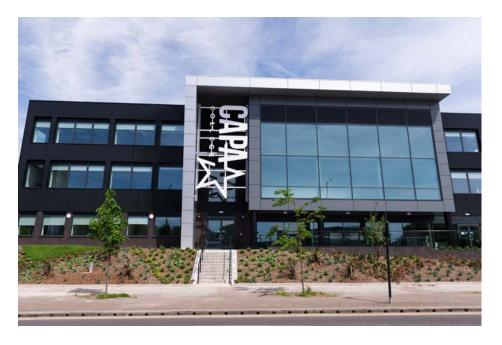
The external built up faceilluminated aluminium logo sign features a 100mm deep rim and return. The LED modules are in a cool white to provide night illumination.
