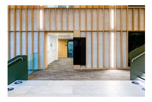
The Jigsaw system uses a secret fixing system to enable the easy changing of panels. It doesn't require a key or any special tools.
