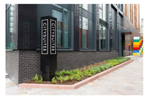
The fabricated illuminated external totem signs are clad with aluminium panels, seamlessly joined. The text detail is stencial cut and inlaid with push through opal lucite.
