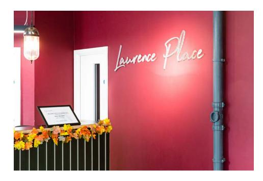
The building name signs use 3mm thick brushed stainless steel with a glass bead blasted edge to provide a superior finish.
