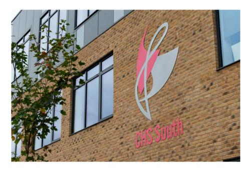
The external CHS logo features a 3mm aluminium logo, coated to match the colour requirements of the scheme. The logo is profile cut and mounted to the external brickwork with suitable wall anchors and adhesive.
