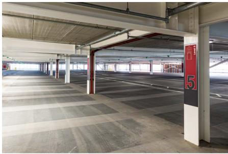
In the car park, a grey band aluminium strip has been mechanically-fixed to columns, with digitally printed vinyl graphics applied to the surface.
