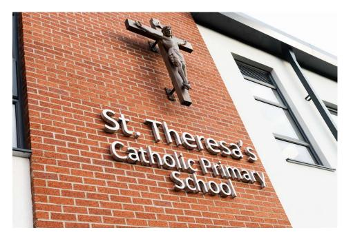
The lettering that features at the front of the building is manufactured from 4mm thickbrushed stainless steel.
