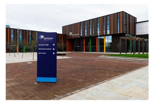
The bespoke aluminium fabricated totems signs with recess edges feature in the courtyard. The totem is fitted to a fundation cage for secure fixing and the panels are texted with self-adhesve vunyl with tamper resistance.
